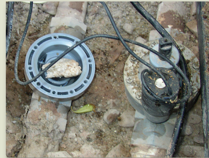
Debris in valves can cause leakage by preventing the valve from closing properly.
